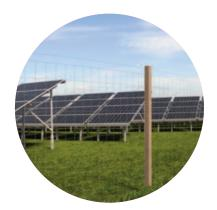
Panels will be mounted individually on a metal frame which is attached to galvanized steel piles that will be driven up to 3m into the ground. The distance between each row of frames is 3.2m - 5m to limit the impact of inter-row shading and there will be a border gap between panels of approximately 10mm to 20mm which will allow rain to pass through.
